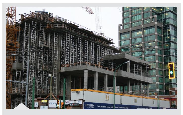
Prefabricated, easily assembled components provide support for slabs, beams and other horizontal formwork.
