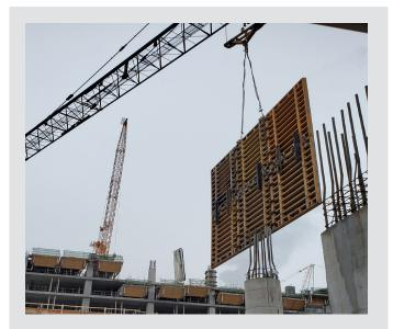
Once the assembly is complete, the gang can be lifted to its final position, with the lifting hooks.
