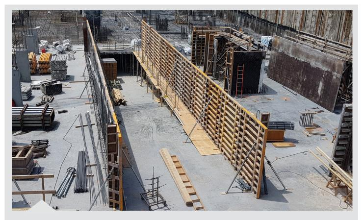
Forming gangs with CLAMPS saves time during assembly because it is possible to set up by simply positioning the panels and tying them with the strike of a hammer. This type of connection allows the panels to be at different elevations because the CLAMPS can be placed anywhere along the panels' perimeter profiles.
