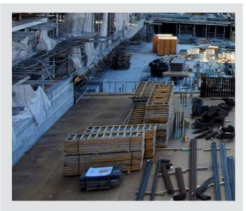
The panls and beams can be moved by crane or forklift and piled up to the height of two pallets. It facilitates the panel/beams' delivery and transport on the building site as well as their erection and later dismantling.
