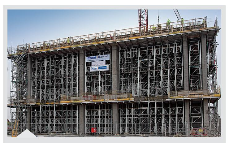
Three basic components with high leg load capacity. 8 point ledger frame connection at same elevation, and platform decks can be fixed onto ledger frames. Integral safe guard-rail with working platform
