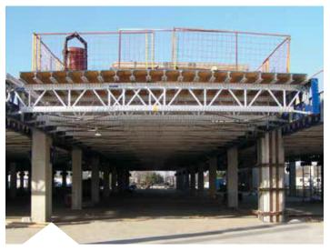
Large trusses can be set to accommodate bay widths up to 31 ft
