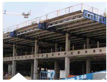
Offsite pre-assembly of major components, reduces job site assembly time
