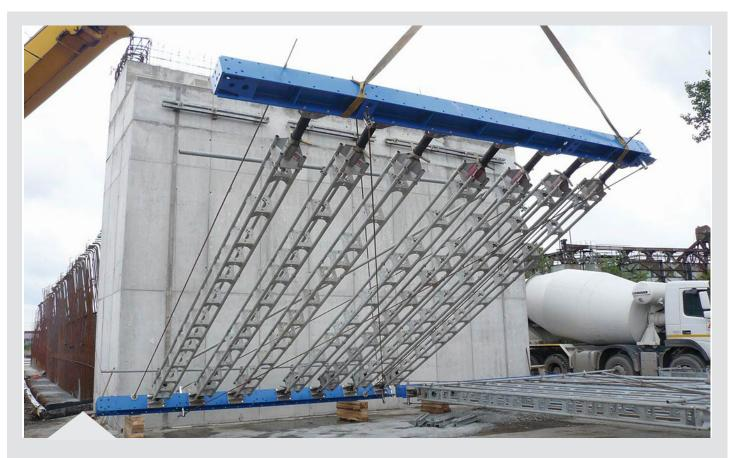
High load capacity thanks to the load-optimised system components. Numerous connections for adapters and compensating connectors enable articulated or rigid connections and increase the variety of shapes to be produced.
