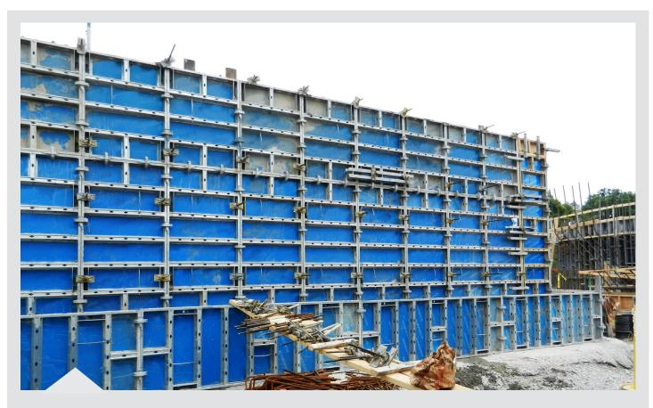
The premise that a quality & affordable handset system should not compromise pour rate, this is how Lite Form was designed. An allowable pour pressure of 1500 psf at any height pour, with a simplistic assembly, makes this system very attractive.
