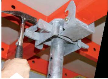
Specially developed folding heads with self-securing pins make it effortless to connect props
