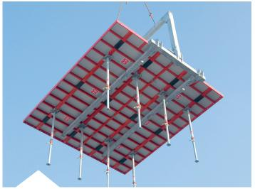
Large forming units up to 26 m<sup>2</sup> transferable in just a single crane pick
