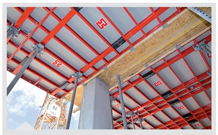
The world's first floor table with a maintenance-free, narrow steel frame combined with plastic form lining. Ideal for the costeffective realization of larger slab formwork projects with regular ground plans.
